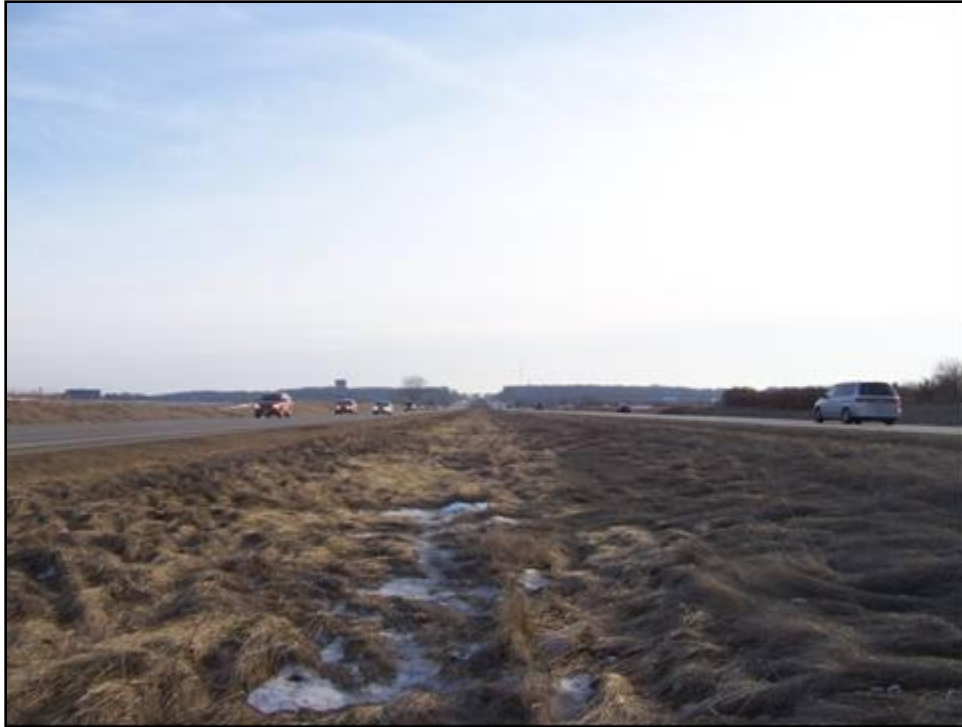
FIGURE 5 Typical Wisconsin Highway Median (I-39 Rock County – 60 feet) (6)
