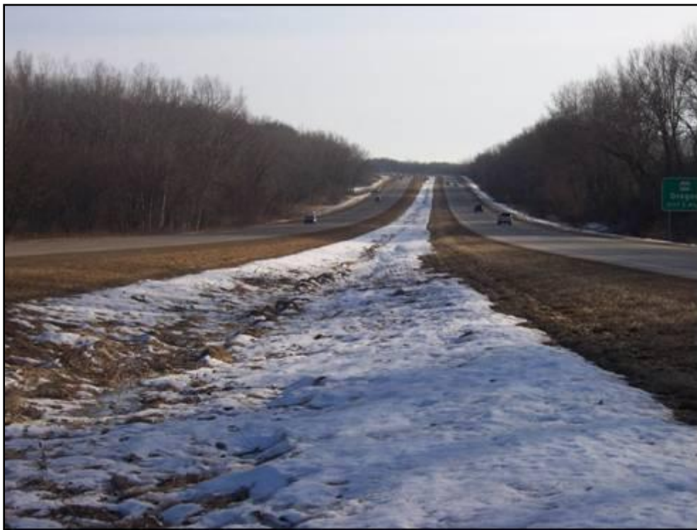
FIGURE 6 Typical Wisconsin Highway Median (USH 14 Dane County – 68 feet) (6)
